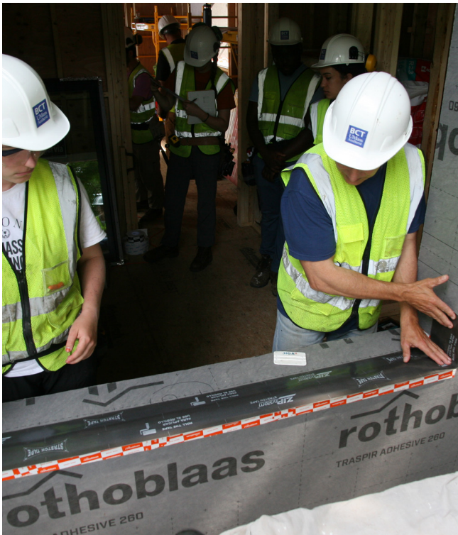
Figure 9. Taping around a window opening.
